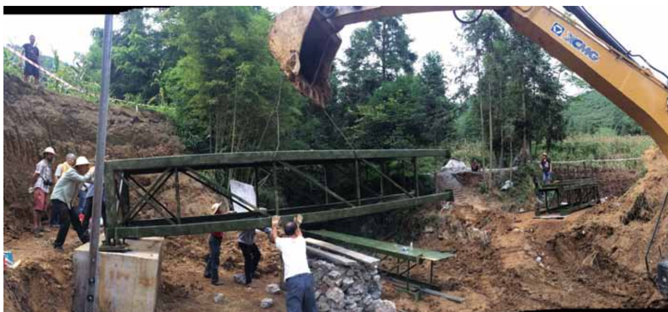
Assembling the footbridge
